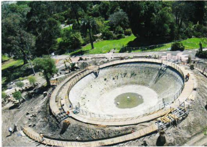
Volcano shell clean, boardwalk and viewing platforms under construction.
