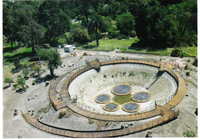
Biofilter disks in place, ready for filling of shell.
