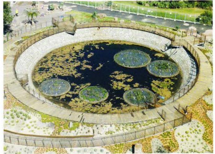
Above: Landscaping advanced, plants growing on biofilter disks. Below: Sign at the site explaining biodisks and their function.
